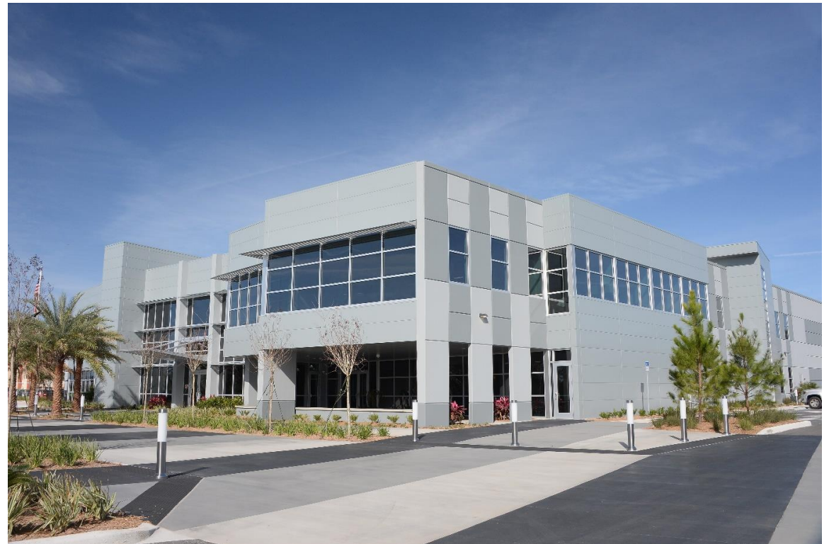
Metrohm, Riverview, FL, HTG Architects, CFA
