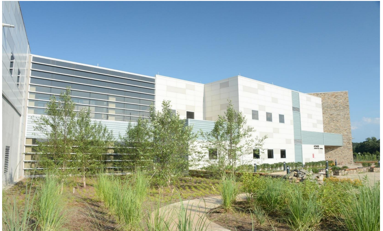
Loudon Water Treatment Facility, Leesburg, VA, CDM Smith
