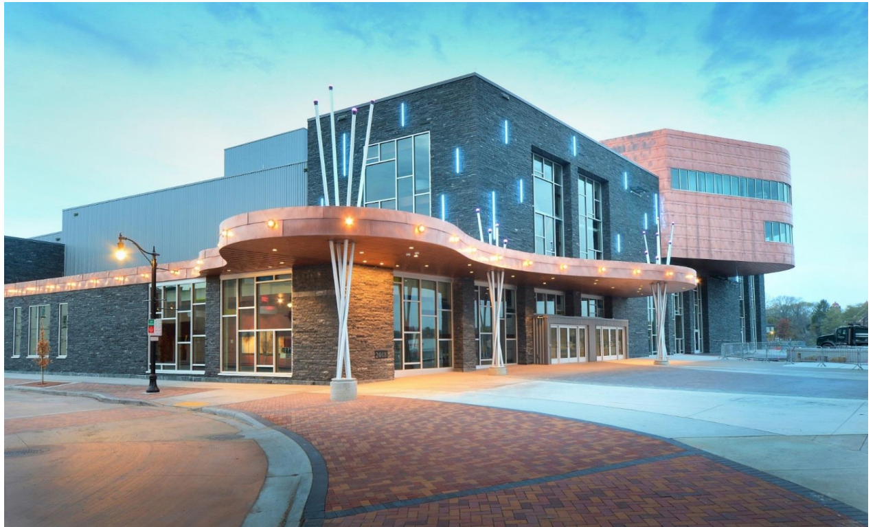
Confluence Center, Eau Claire, WI, Holzman Moss Bottino Architects
